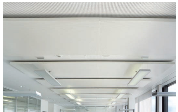
Fig. 6: Multifunctional sails pushed over the traverses
